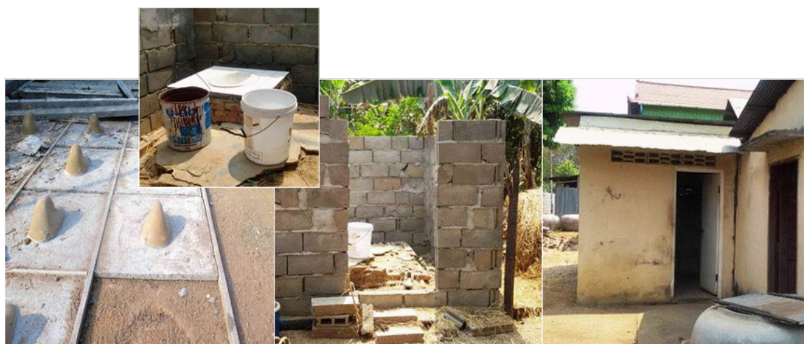
Concrete toilet slab production centre
