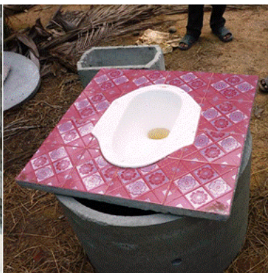
Pour-flush toilet slab ready to be installed and used
