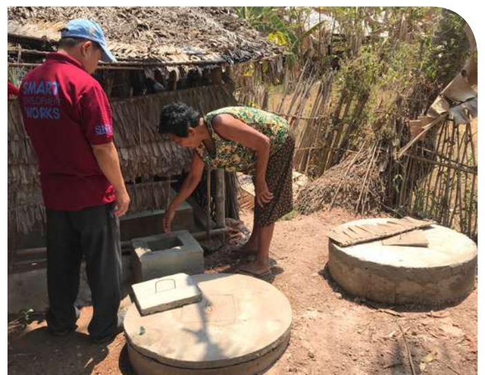
Figure 4 – Inspecting a newly constructed Alternating Twin-Pit latrine
