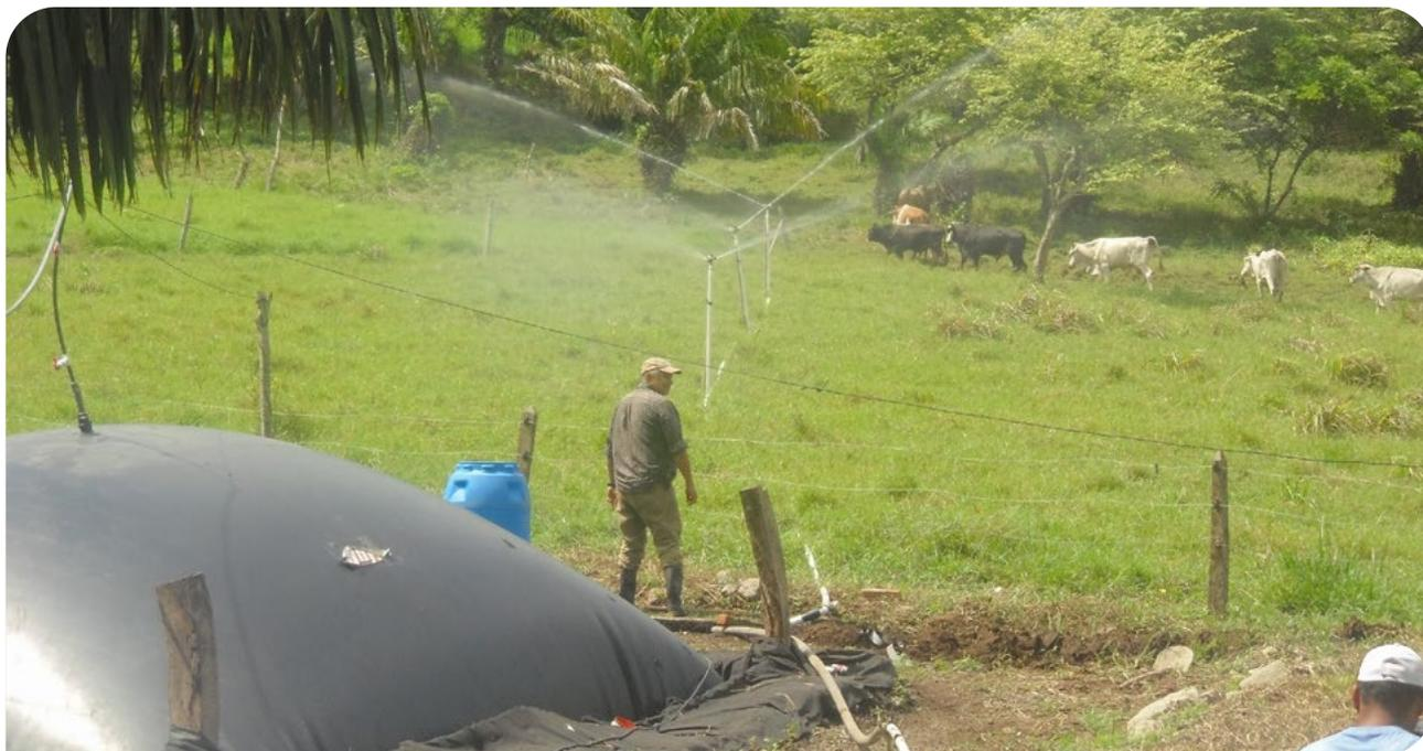
Productive use of biogas from a medium-scale biodigester for sprinkler irrigation in Nicaragua.
