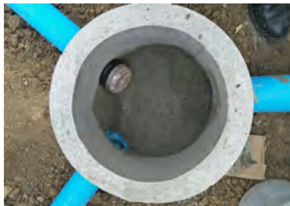
Figure 1 – Alternating twin-pit and diversion box configuration
