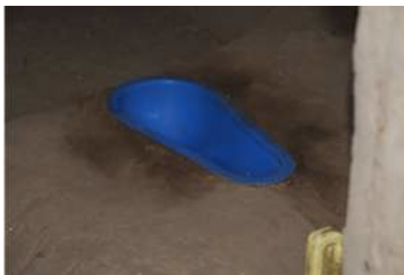
Figure 20: SATO pan installed in a village household latrine
