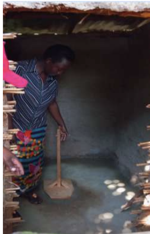
Figure 17: An improved facility with drop hole cover
