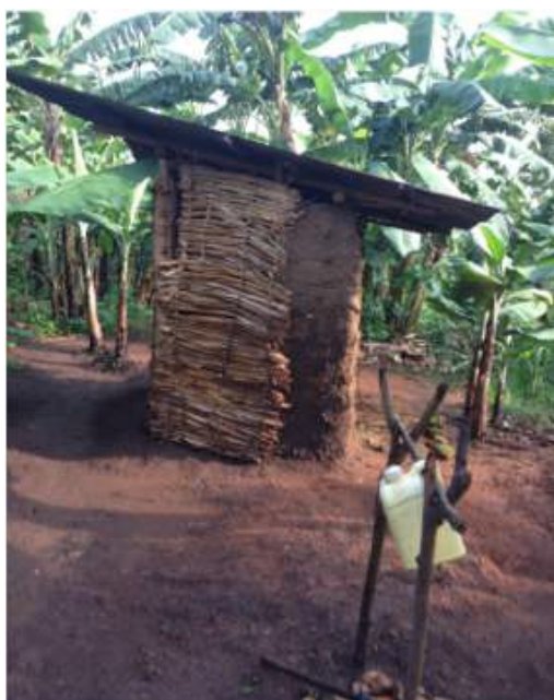
Figure 10: A well built latrine with HWWS facility in Kibende village, 2017.
