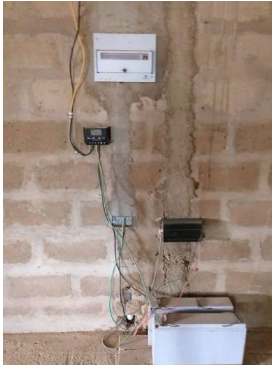
Solar systems connection in one of the households
