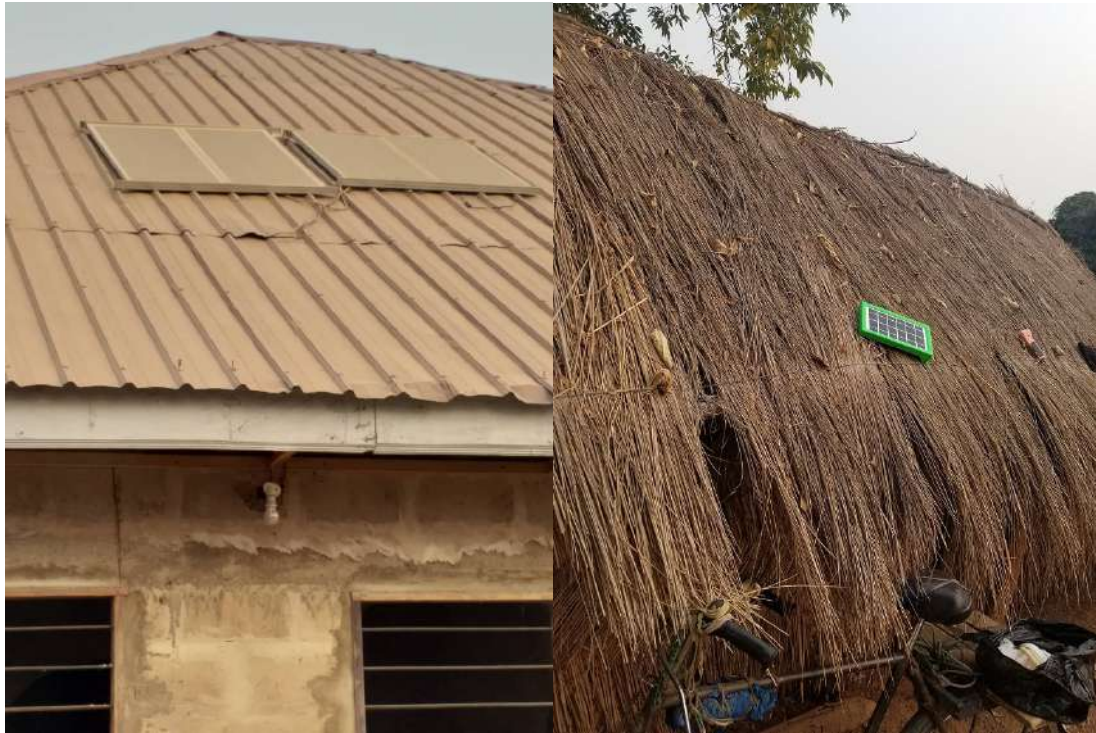
Figure 2: PV Panels for charging lanterns and home systems
