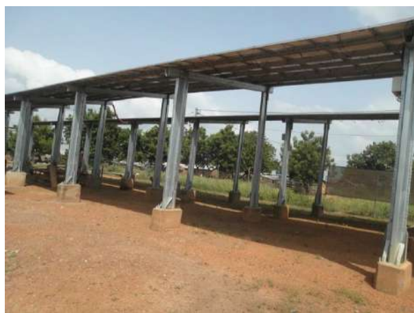
Figure 4 Solar module infrastructure at Kudorkope
