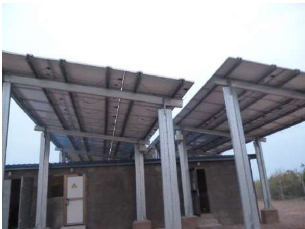
Figure 9 Solar module infrastructure at Aglakorpe
