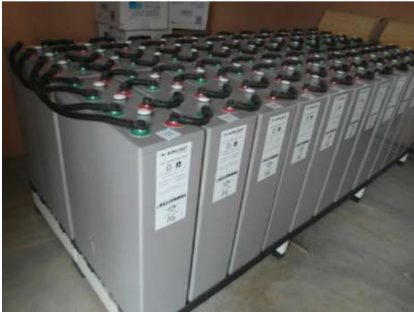
Figure 5 Solar battery bank at Kudorkope
