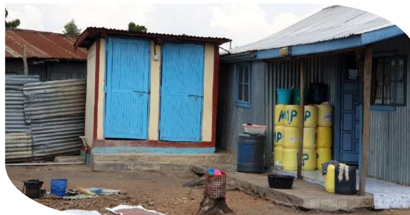
Toilet unit constructed in Shauri Yako slum area. Photo by ADRES Group.
