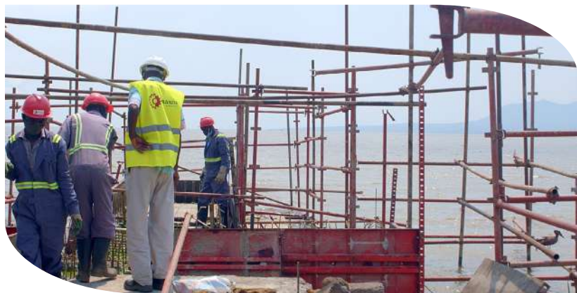
Construction of a new water storage facility to increase clean water supply in Homa Bay. Photo by ADRES Group.
