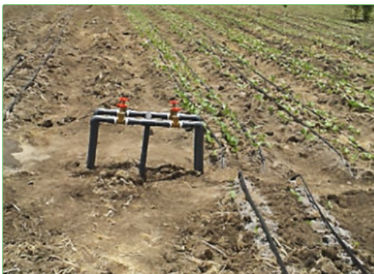
A system of main pipe joining a tee junction that distributes water to the sub main lines on both sides.
