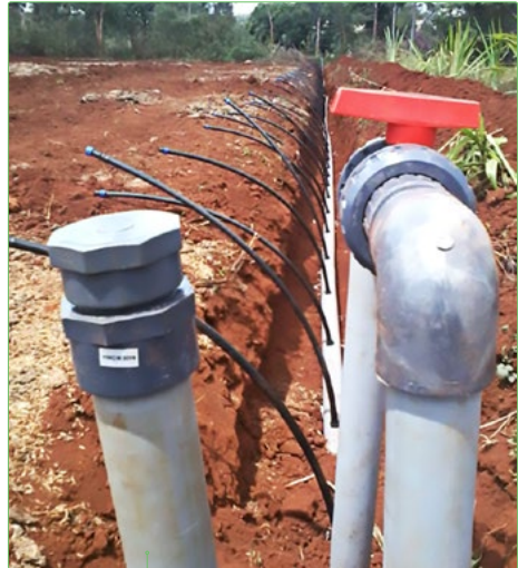
A Lateral composed of pipe risers that will be connected to the driplines and a ball valve that controls the flow into the lateral.
