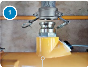
1 Hydraulic connection: standard camlock connectors for easy and tight fit.
