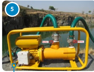
5 Hoses connected to the pump
