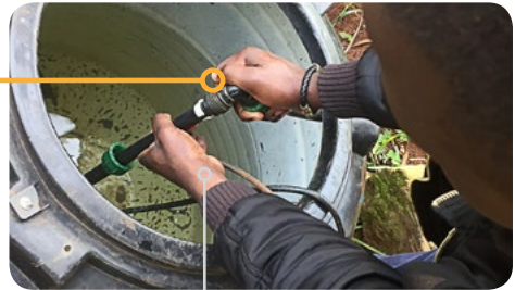
connection from pump to outlet sprinkler or drip kit.
