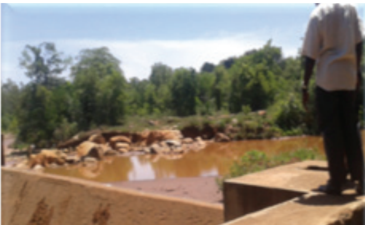
Kanyadhiang water project was completed in 2012 by LVSWB with KSh.123 million investments from Dutch government. The project was to benefit 19,000 men and women of Kanyadhiang village in Homabay County. Within 3 years of completion, the project stopped functioning due to siltation and breakdown of river intake structure, wasting all the investments made. SNV has been supporting the WUA to engage a private firm to manage the water system.
