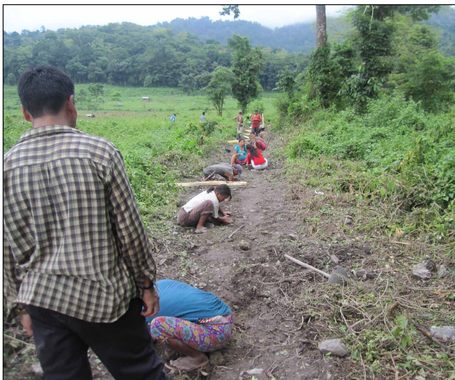
ToT on Human-wildlife Conflict Management through Electric fencing at Sershong, Tashiphu. Farmers' participation for digging holes for fixing poles
