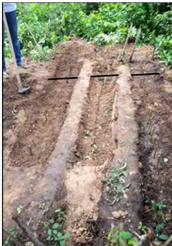
Figure 12. Trenches dug for burial of faecal sludge. (Photo: Wetlands Work)
