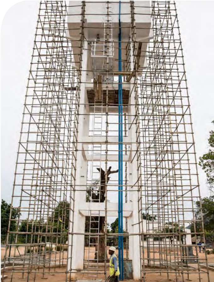
Photo: Building a community water supply tower in Mozambique (SNV/PRONASAR).
