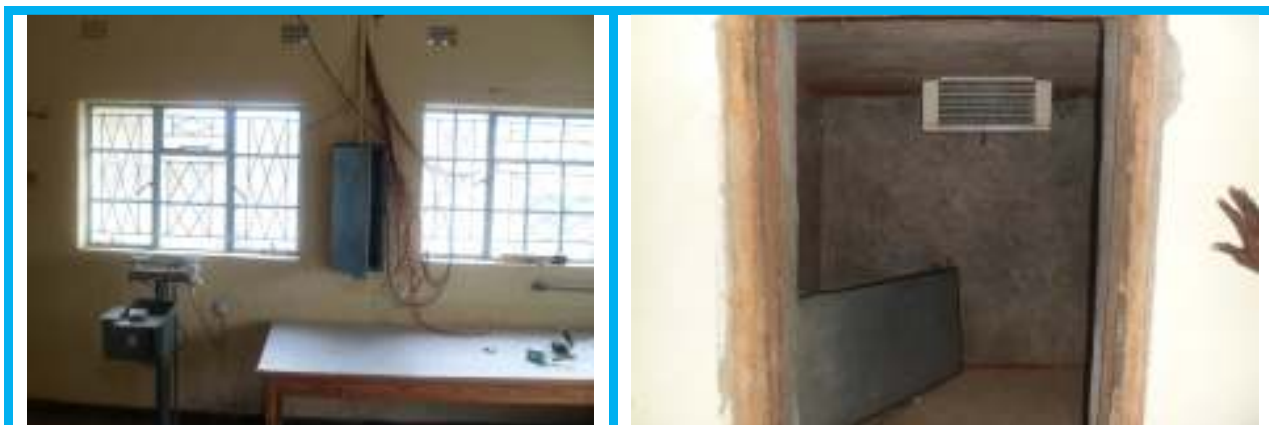
Illustrations: Highlights of key renovations and equipment repairs before business resumption.
