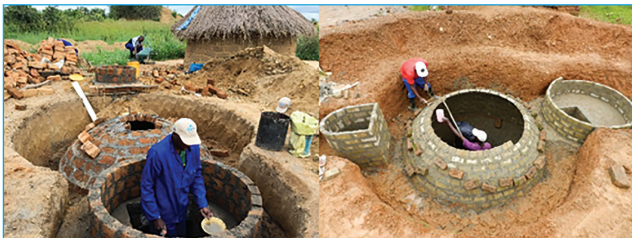
EXHIBIT 1: CONSTRUCTION OF FIXED DOME BIODIGESTERS
