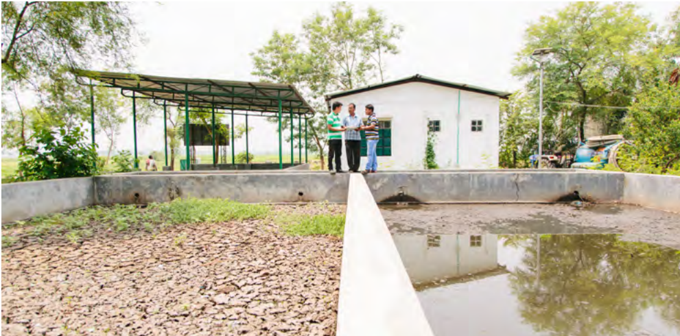
Sludge drying beds at the Kushtia FSTP
