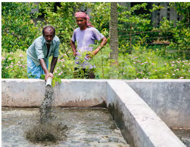
Discharging sludge into drying beds
