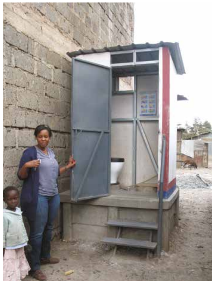
The SafiSan pour-flush toilet model adopted by Tharaka Nithi County. The model was introduced by Water Sector Trust Fund to improve sanitation in water-scarce areas
