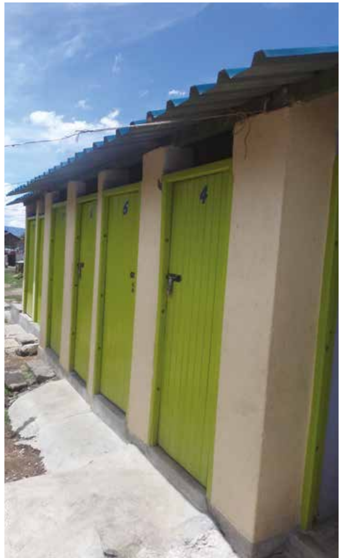
County housing sanitation blocks - after rehabilitation
