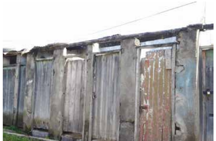
County housing sanitation blocks - before rehabilitation
