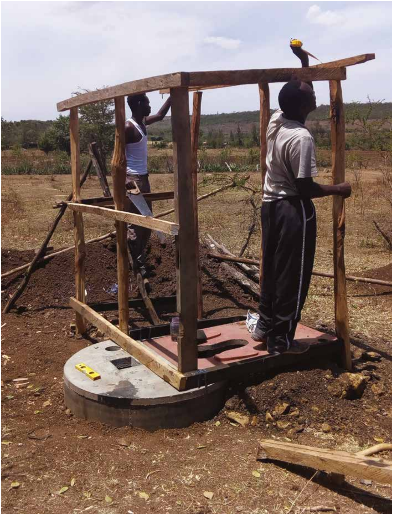
SAFI latrine installation
