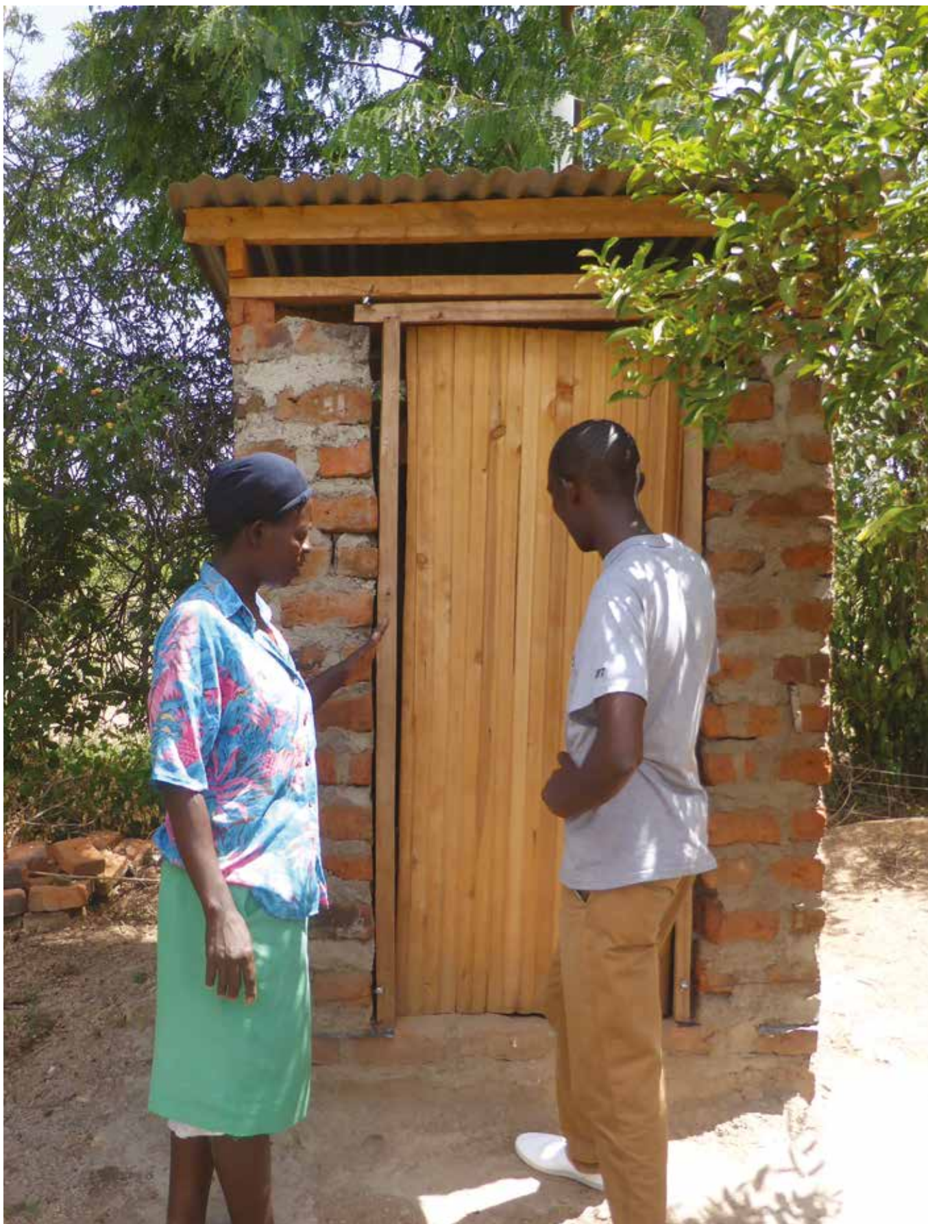
Toilet facilities in use
