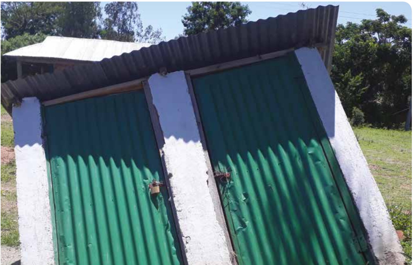
A collapsed latrine in Wang'chieng
