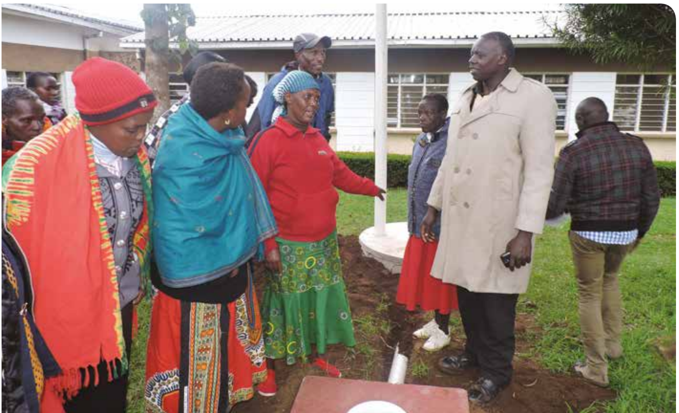
SAFI latrine Demo site installation in Kaptarakwa ward
