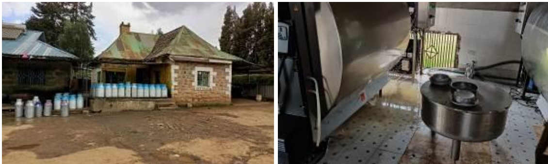
Figure 17: External View of dairy (left), inside the dairy plant (right)
