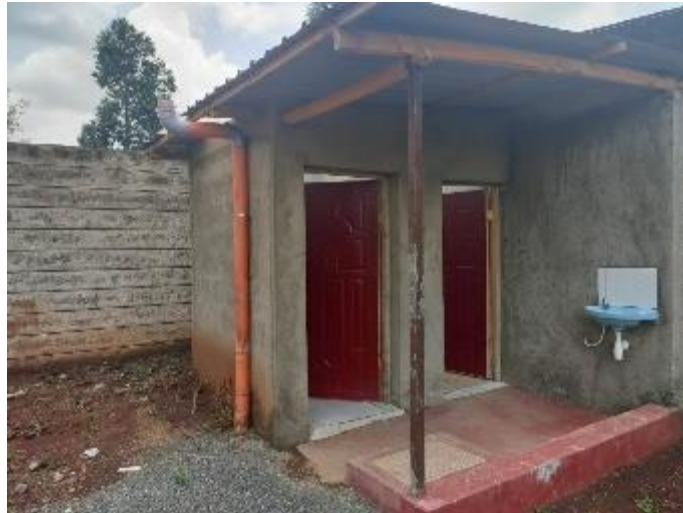
Figure 13: One of the toilets at the factory
