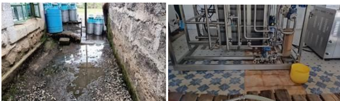
Figure 18: Poorly managed milk container facility (left); machine not yet installed (right)
