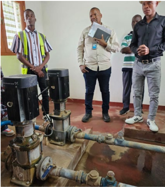
Photo: Pumping water to an elevated tank
