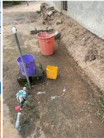
Photo: A typical household connection
