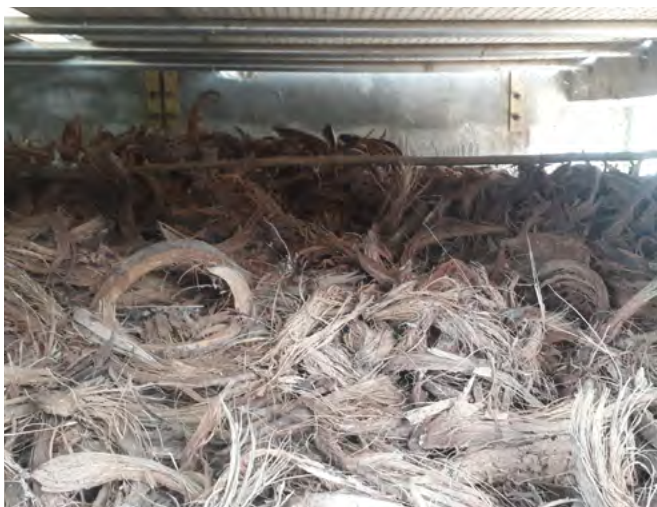
Filtering effluent in coconut dust and coir filtering bed
