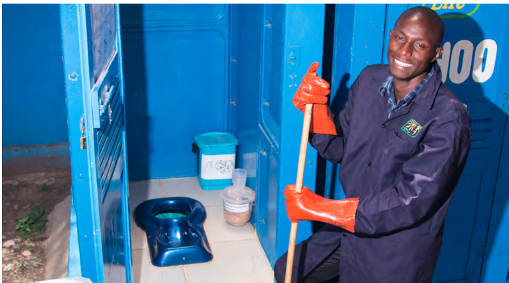
Fresh Life container based, urine-diverting toilet
