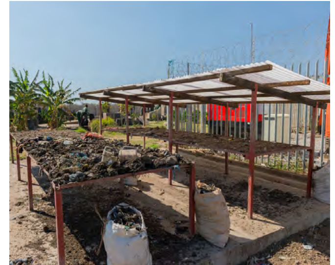
Sorting and drying solid waste at Kanyama FSTP
