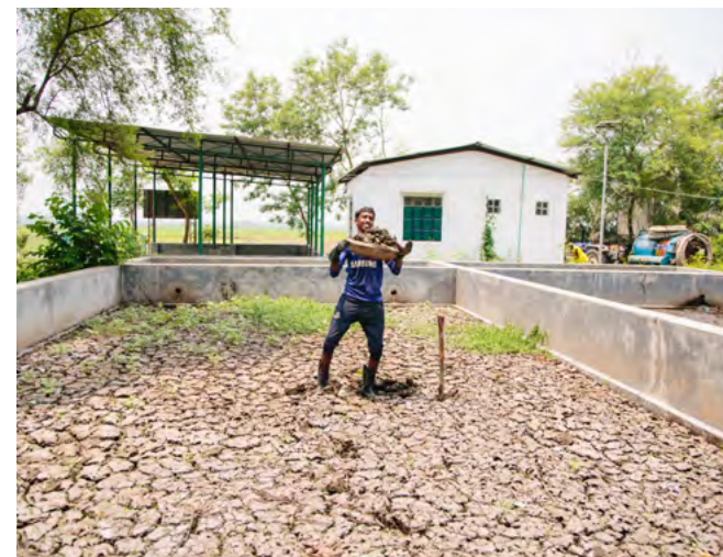
Removing dried sludge from the drying beds
