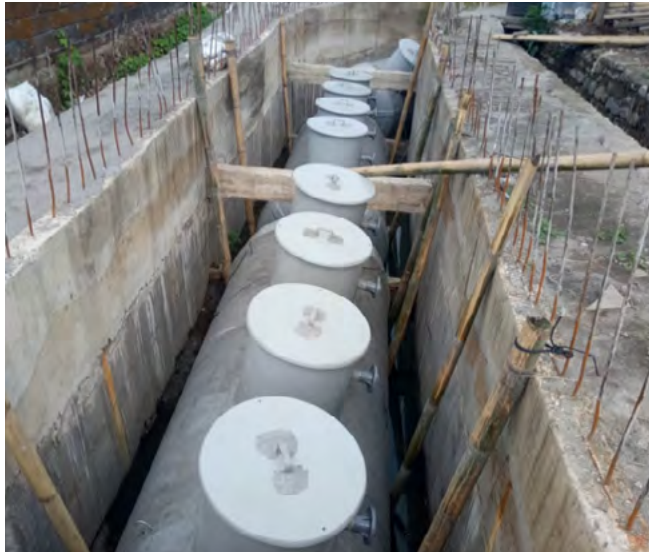
Installation of DEWATS technology
