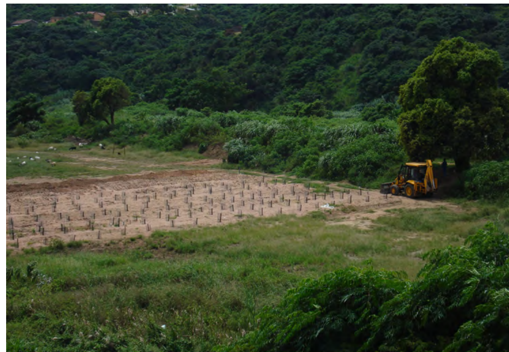
Umlazi planted trenches site in South Africa
