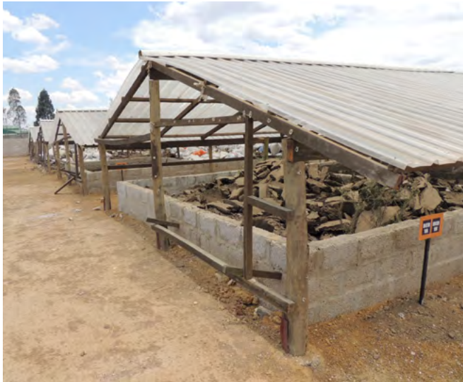
Roofed sludge drying beds at Kanyama FSTP
