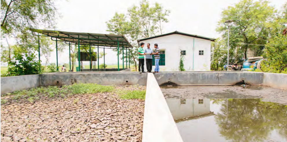
Sludge drying beds at the Kushtia FSTP
