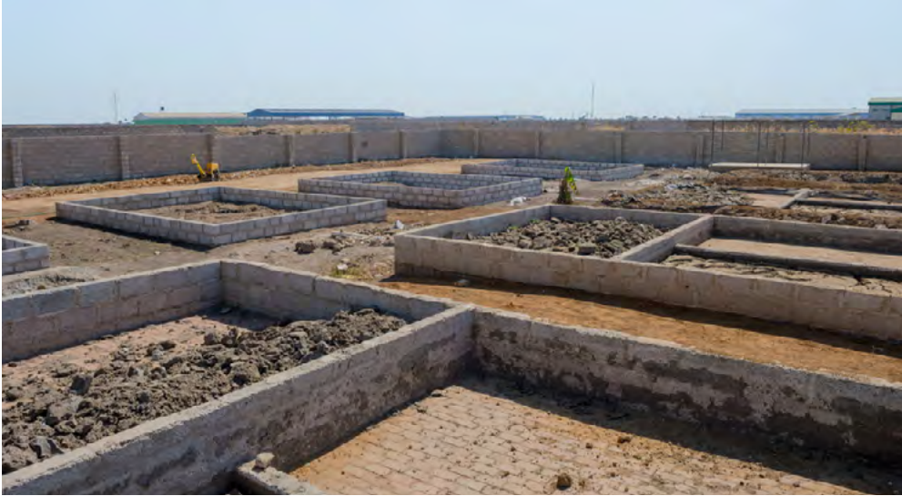
Kanyama FSTP decommissioned sludge drying beds
