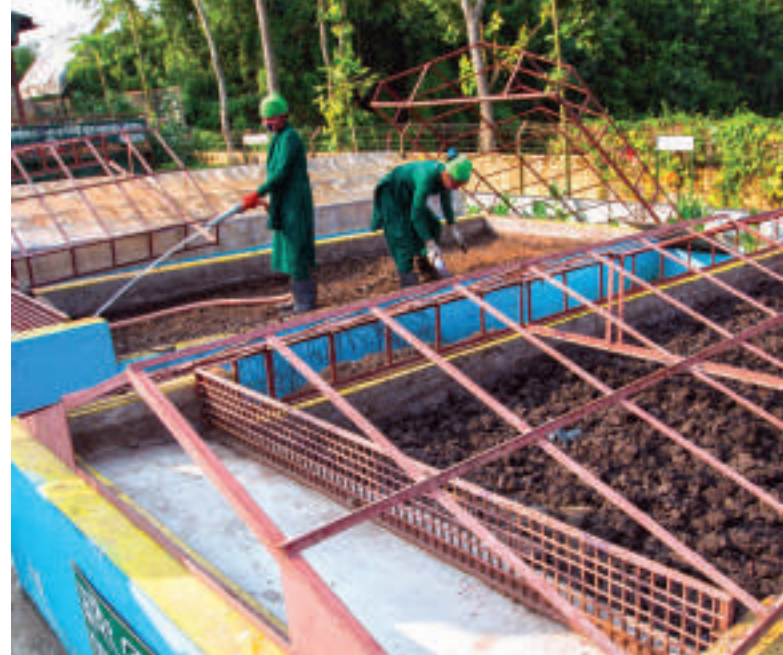
Two works of Sakhipur co-compost plant preparing the drying bed
