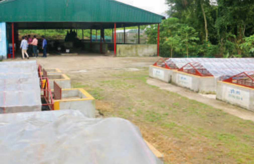
The plant is operating for the last two and half year and treated approximately 2400 MT faecal sludge and 250 MT solid waste.
