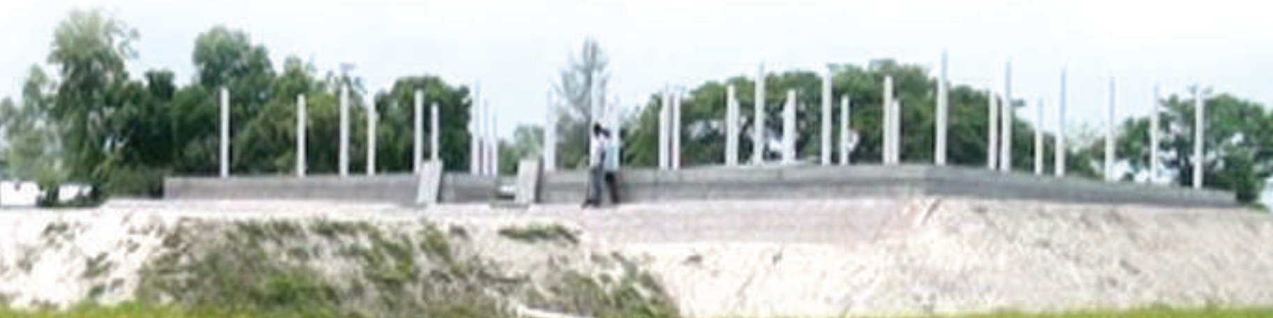
Construction work of the faecal sludge treatment plant in Sirajganj municipality
