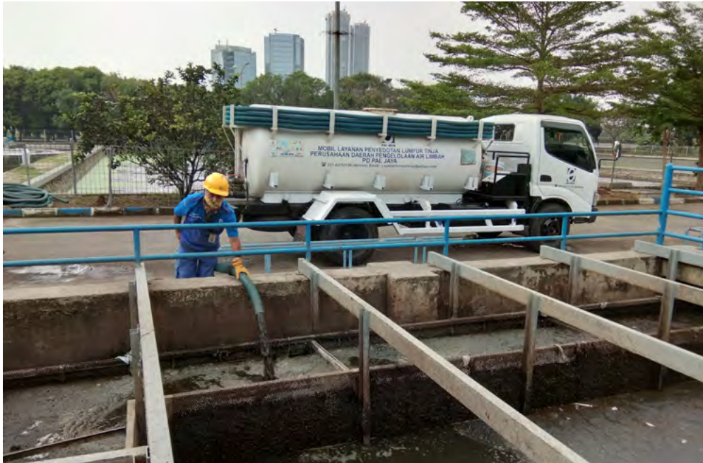
Conventional aerobic pond
