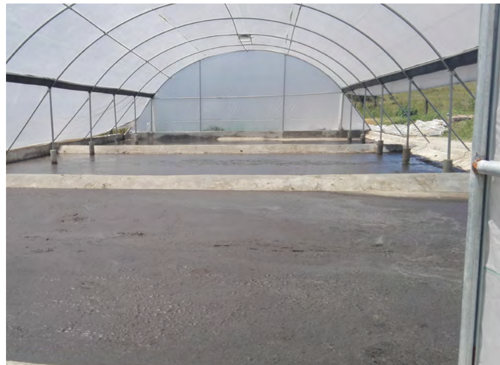
Solar dryer in the NAWASSCOAL facility
