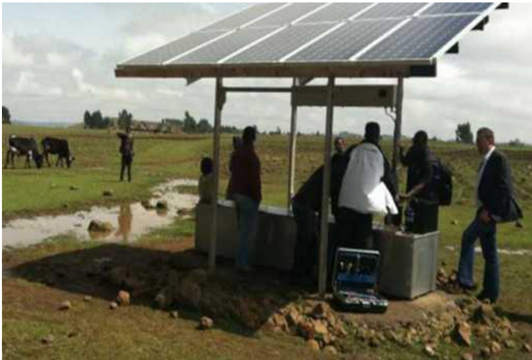
Figure 3: Solar powered milk cooler
